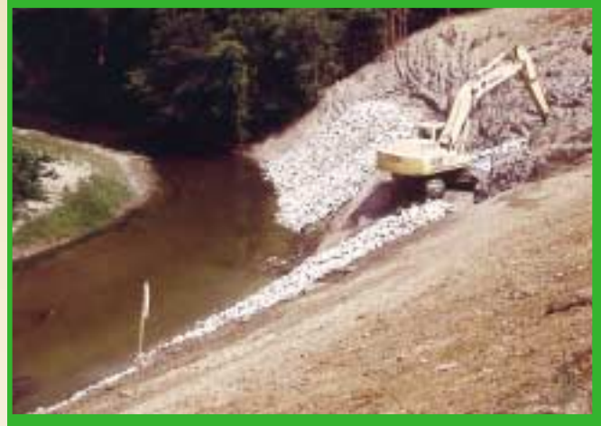
White Lick Creek stabilization at Timber Bend subdivision. 1997.
