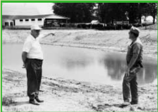
N.C. Brown (left) and Conservation Technician David Sowers look over a new animal waste holding pond. 1973.
