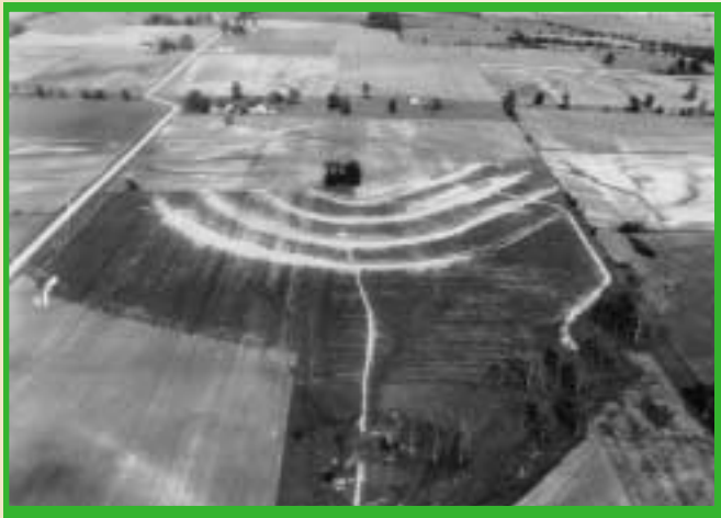
Partially completed parallel tile outlet terraces on Melvin Buescher farm. 1961.
