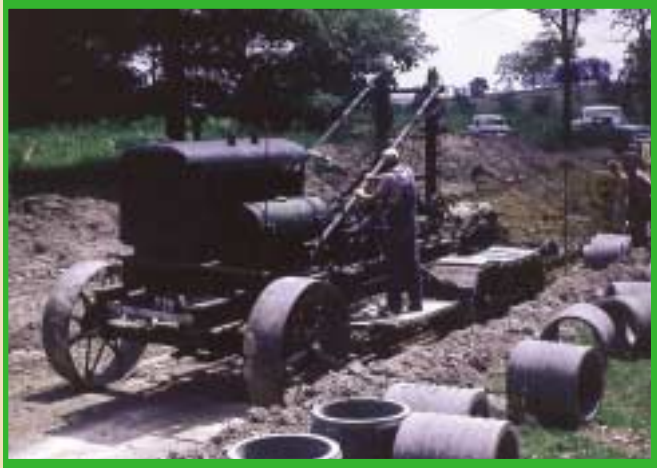
Travis-Prichett Group Tile Project. Contractor Sam Dickerson purchased tile machine especially for this 20-inch tile project. Early '60s.
