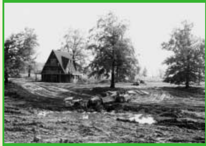
Harold Hiser's pond under construction.
