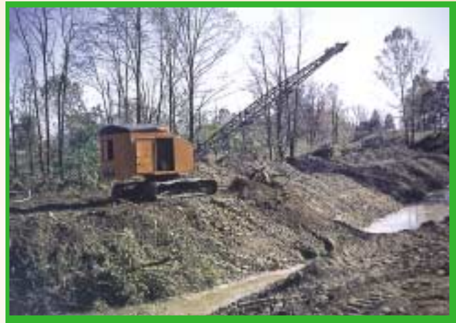
Barnett Ditch reconstruction 1958-'59.
